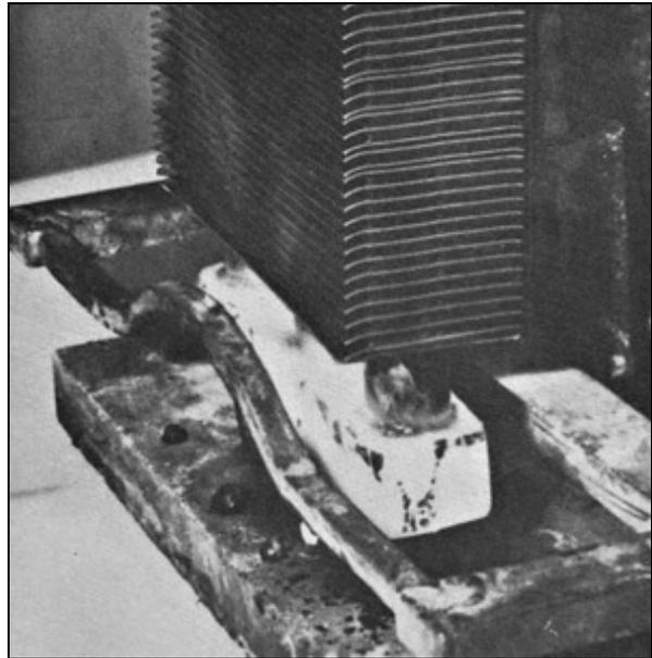
Figure 5: Copper sheet is induction brazed to 100 small tubes, and simultaneously, to the housing of marine coolers
